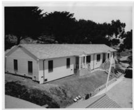
Another view of the modern Duplex under construction, 1960.
