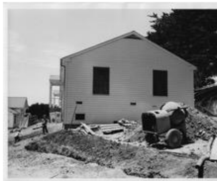
Children playing at the new Duplex's construction site – most likely Eric and Gail Settlemier, son and daughter of Robin "Bob" Settlemier, Coast Guard officer-in-charge 1959-1960.
