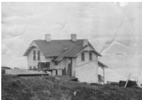
Double Keepers Dwelling under construction, 1890.
