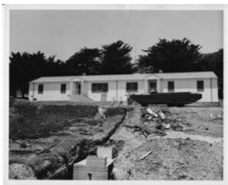
Modern Duplex under construction with "duck" in front, 1960.
